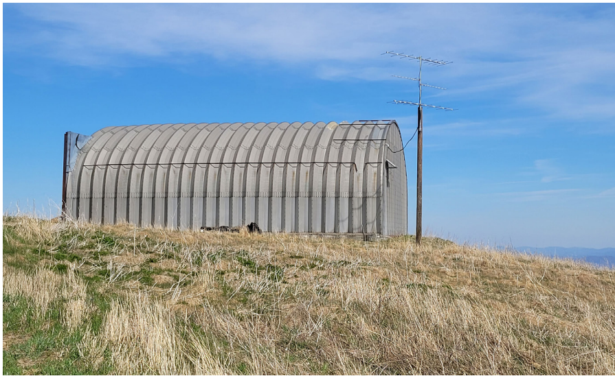
The Pond Mountain Motus Station in Ashe Co, NC. Antennas are mounted on a wood utility pole and the station's battery is charged by a solar panel. The receiver box and battery are housed inside this old airplane hangar. (Chris Kelly)
