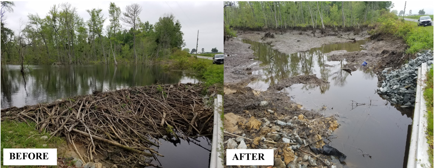
Joey Smith USDA Wildlife Services—Herman Lane Road, Wayne County, May 5 and 13, 2022. A beaver dam built in front of a DOT culvert was pushing water onto the road’s shoulder and threatening its structural integrity. BMAPS’s beaver damage management activities restored normal water drainage, preventing damage to the roadway, saving nearby timber, and protecting the driving public.
