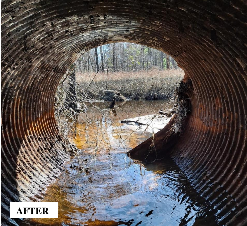
Reid Cooper, USDA Wildlife Services — Beasley Mill Road, Duplin County, February 15, 2023. A beaver dam blocking a DOT culvert was threatening its structural integrity and causing roadway flooding. BMAP services restored normal water flow, preventing damage to the roadway, saving nearby timber, and protecting the driving public.
