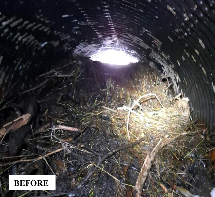
Reid Cooper, USDA Wildlife Services — Beasley Mill Road, Duplin County, February 15, 2023. A beaver dam blocking a DOT culvert was threatening its structural integrity and causing roadway flooding. BMAP services restored normal water flow, preventing damage to the roadway, saving nearby timber, and protecting the driving public.
