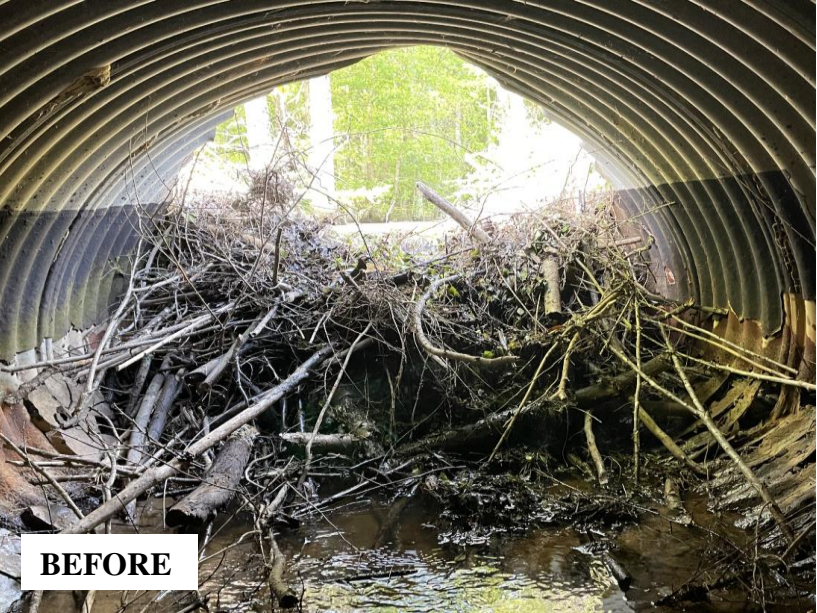
Nicholas Ryan USDA Wildlife Services—Benson Hardee Road, Johnston County, May 12, 2023. A large culvert was in the process of being blocked by beavers. BMAP services prevented further blockage and restored normal water drainage, protecting the driving public as well as prevented adjacent timber stands from being impacted, benefitting multiple adjacent landholders.
